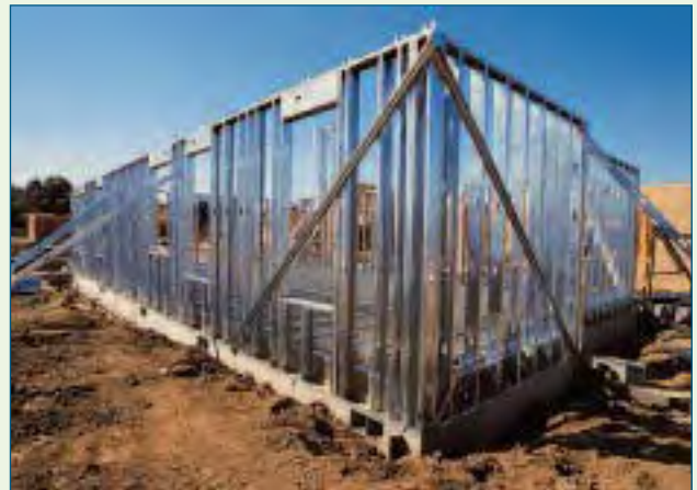
figure co.9 The zinc coating of galvanised steel house frames protects the steel in two ways: it forms a barrier that prevents oxygen from reaching the surface of the steel and also it is oxidised in preference to the steel due to its greater reactivity.
