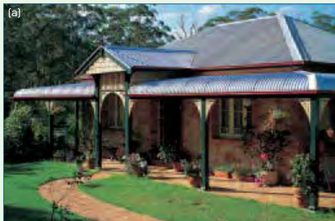
figure co.11 (a) Galvanised iron roofs are common throughout Australia. (b) The iron is protected as the zinc coating gives up its electrons.
