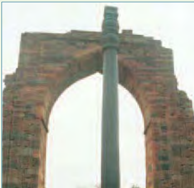
figure co.7 This 1500-year-old pillar in Delhi shows little signs of rust due to the high purity of iron from which it is made.
